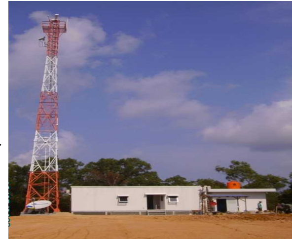
RCC / REGIONAL CONTROL CENTER →
