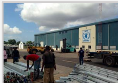
UNHRD facilities in Accra and Las Palmas served as regional staging areas and the Accra depot hosted UNMEER headquarters.
