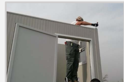
In collaboration with WHO, UNHRD began procuring and dispatching equipment to establish camps for teams tracing EVD. The RRT are building the camps.
