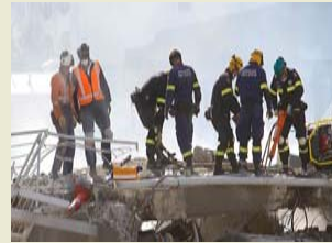
New Zealand 2011 Earthquake
