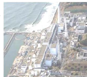
Fukushima Daiichi Nuclear Power Station
