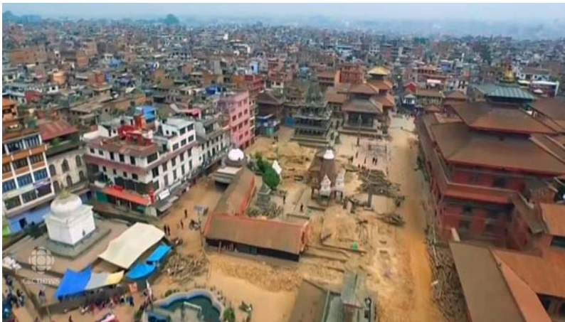
Image taken by a drone after the April 2015 Nepal earthquake
