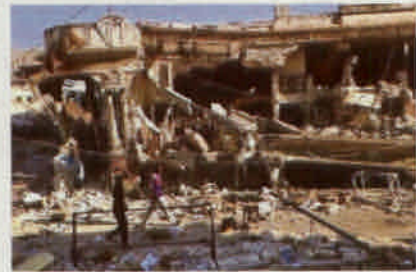
Earthquake in Haiti (2010)
